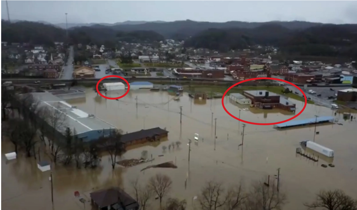
Figure 74: Richlands EMS and Police Station during the February 2020 Floods
